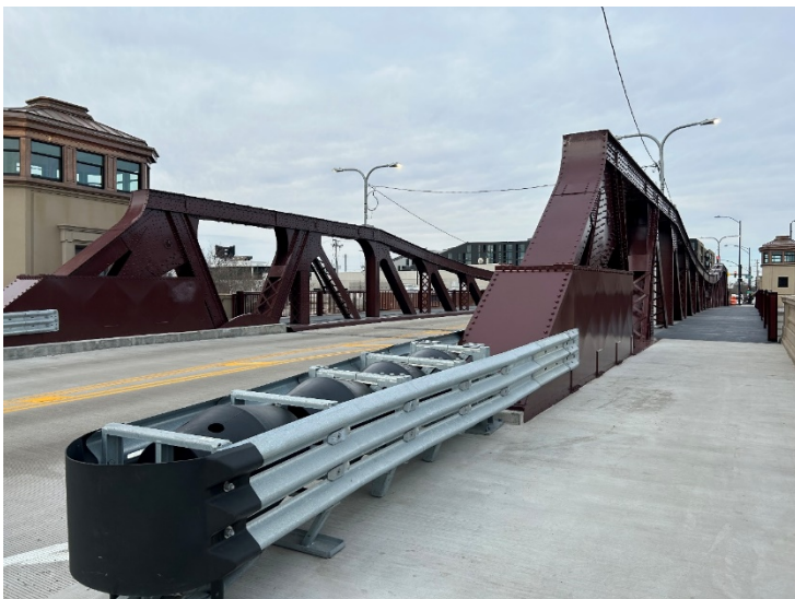
Newly rehabilitated Webster St Bridge over the Chicago River
